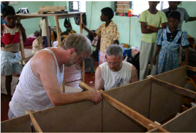
Mike &amp; Steve building shelves at Arudpany
