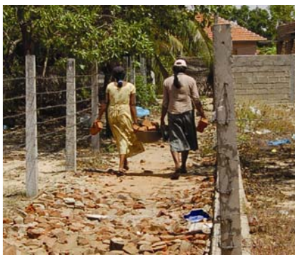
Women carry bricks to build the toilet.
